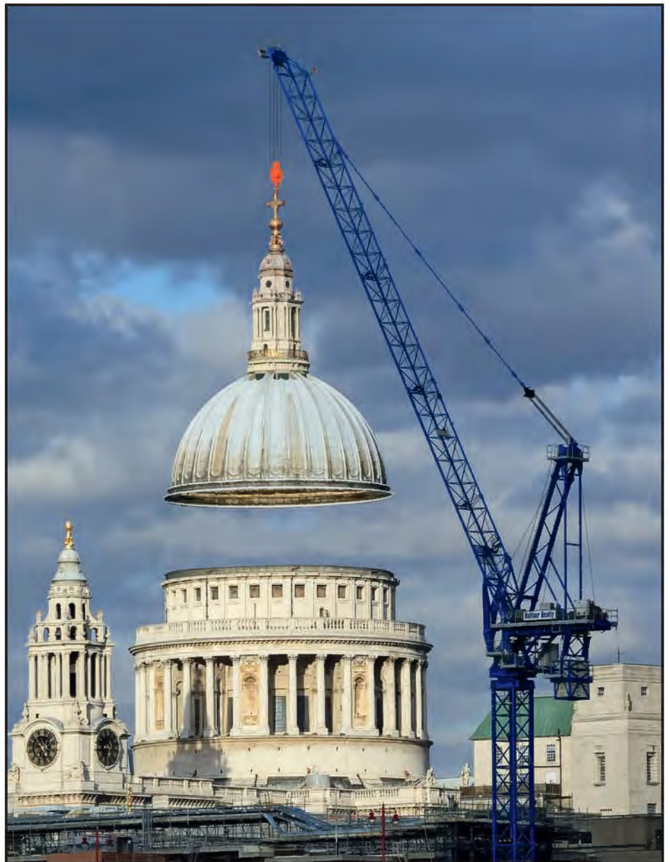
Raising the Roof
