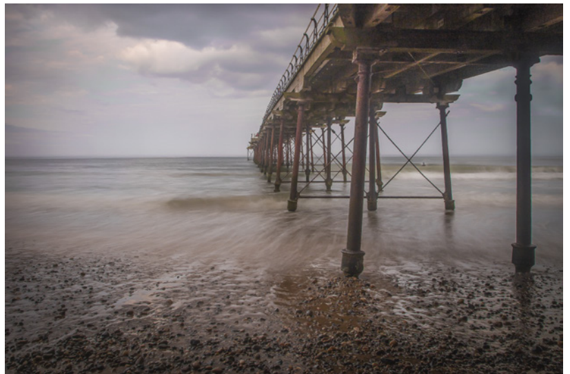
"On the Pier" - Andy Pinch LRPS
