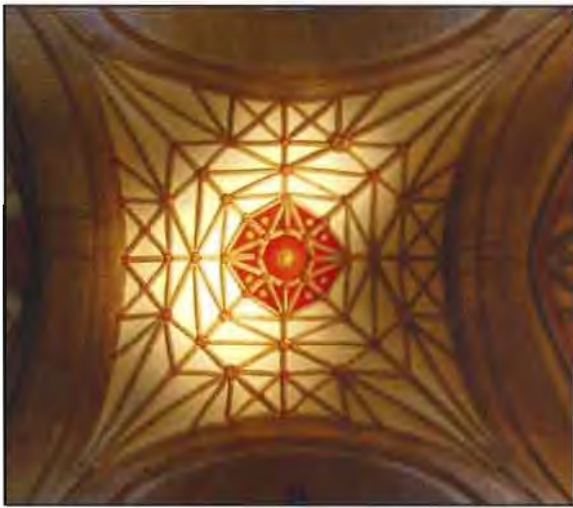
Chancel Ceiling Tewksbury Abbey
