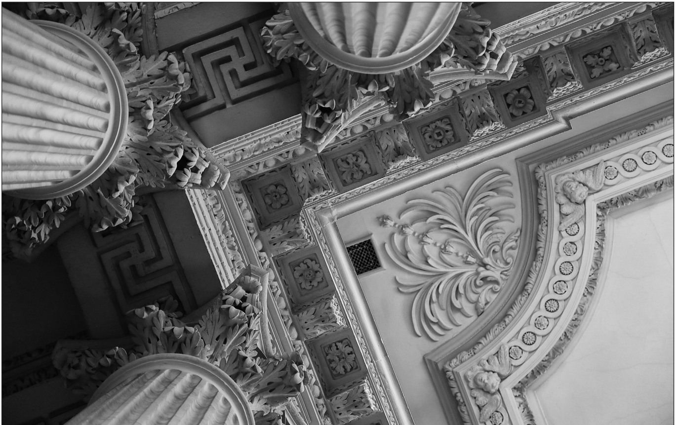
Roof detail at St Vedast, London
