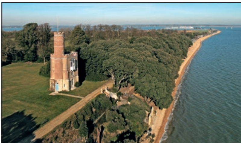
Luttrell's Tower, Southampton, Hampshire
