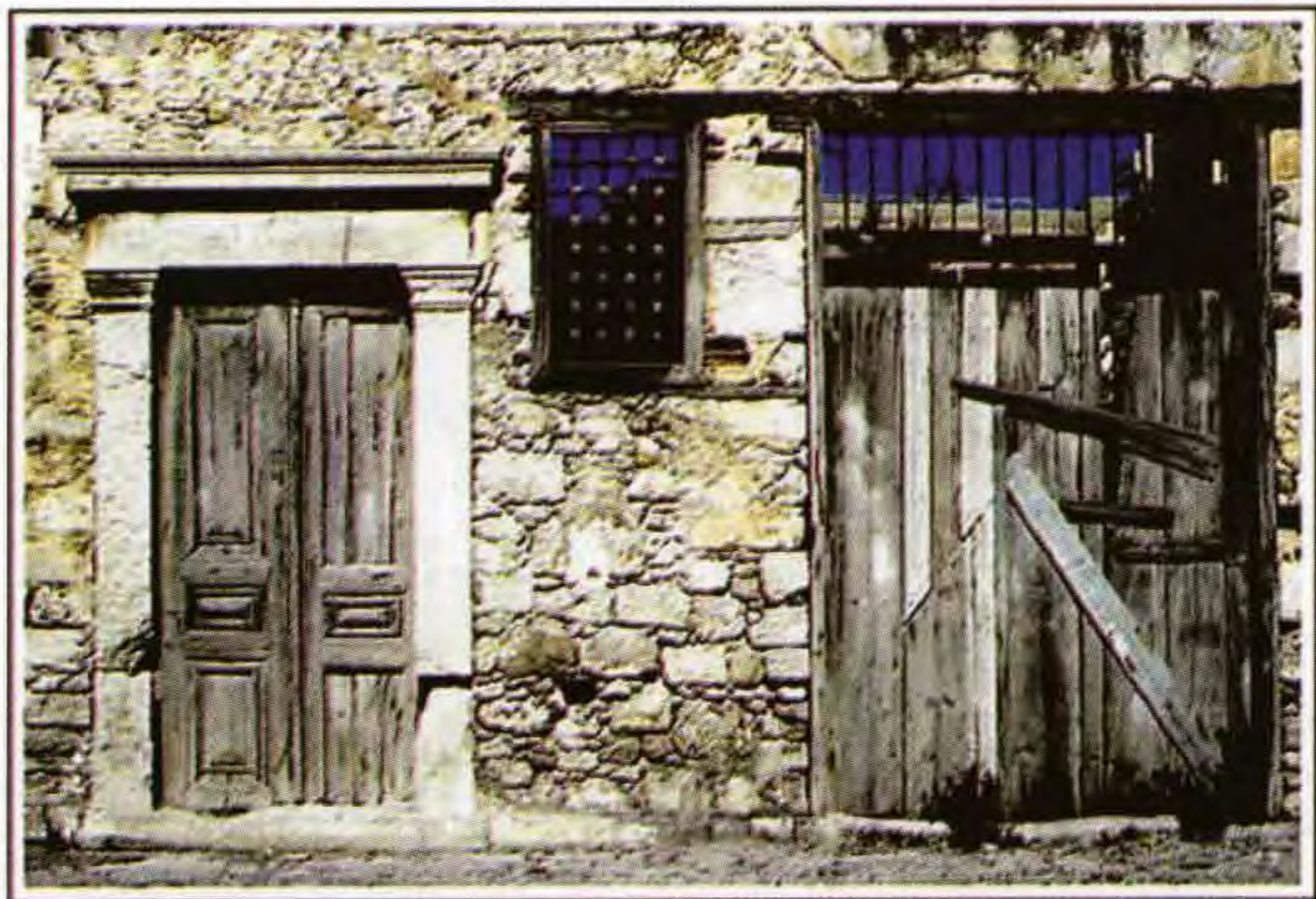
Window and doors
