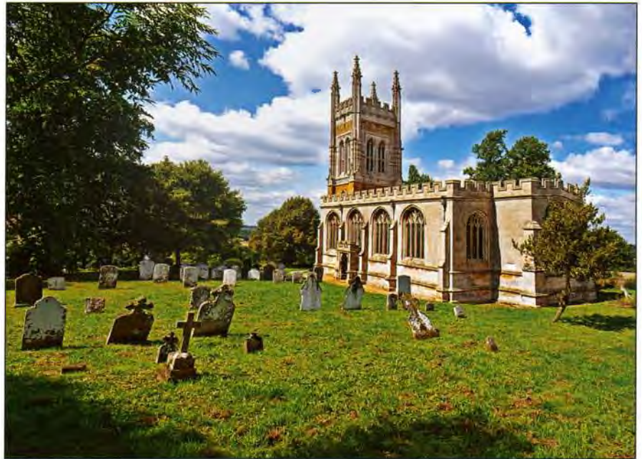
Whiston Church, Northamptonshire
