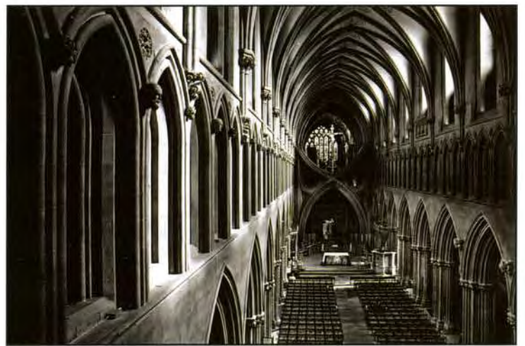
Scissor arch in nave
